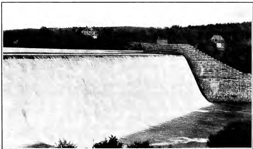
B. DAM ON CHICOPEE RIVER AT RED BRIDGE, MASS., AUGUST 30, 1914.
